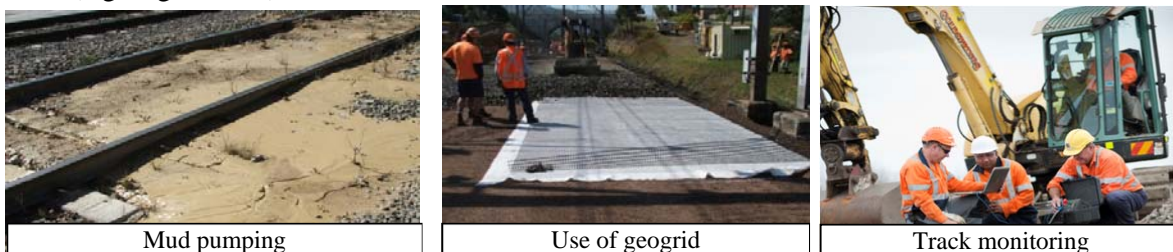
Fig 2. CGRE research involving mud pumping, ballasted rail track improvement through the use of geogrids and real time performance monitoring.
